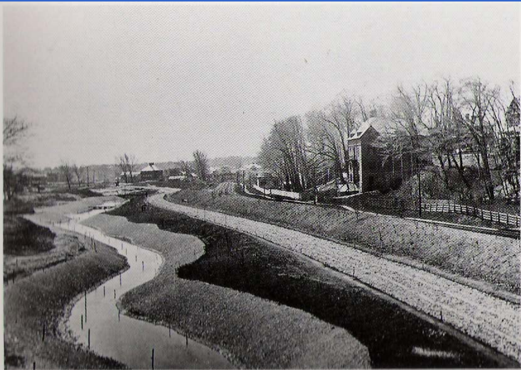
Riverway under construction, c. 1892.
